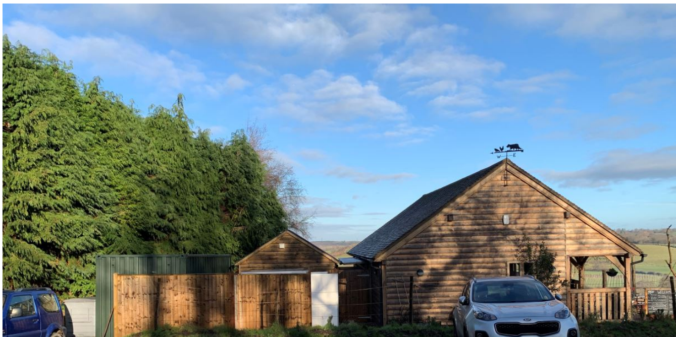
Side of premises showing boundary of neighbouring property (fence and leylandii trees) - Tibbs Oasthouse
